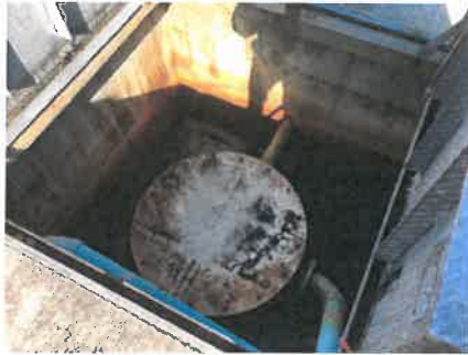
#10: Acid reduction tank (1)
