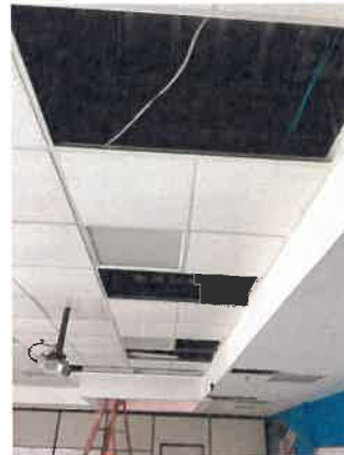
#4 cont'd: Skylight renovations without barriers.
