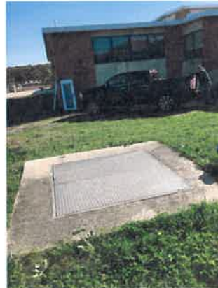
#9: Acid reduction tank grade to adjacent building.
