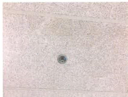
#22: Ceiling outside jr/sr cafeteria.
