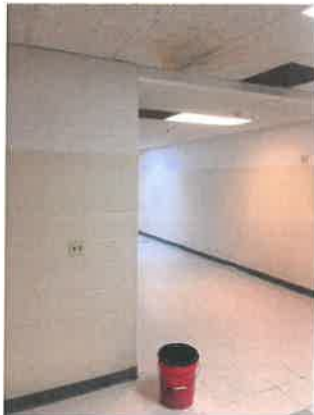
#18: Hallway ceiling 1700 next to elevator.
